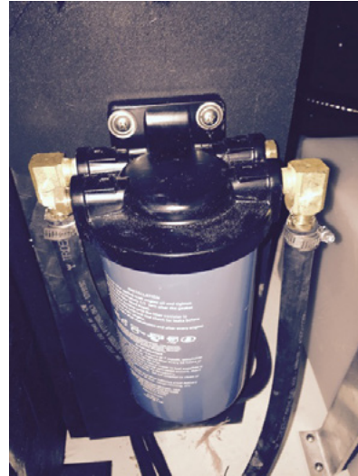
CHECKING IN-LINE WATER SEPARATOR FILTER
