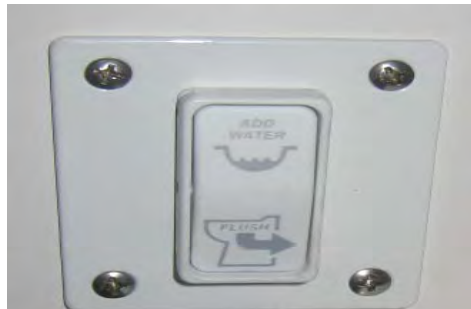
TYPICAL HEAD WALL SWITCH
