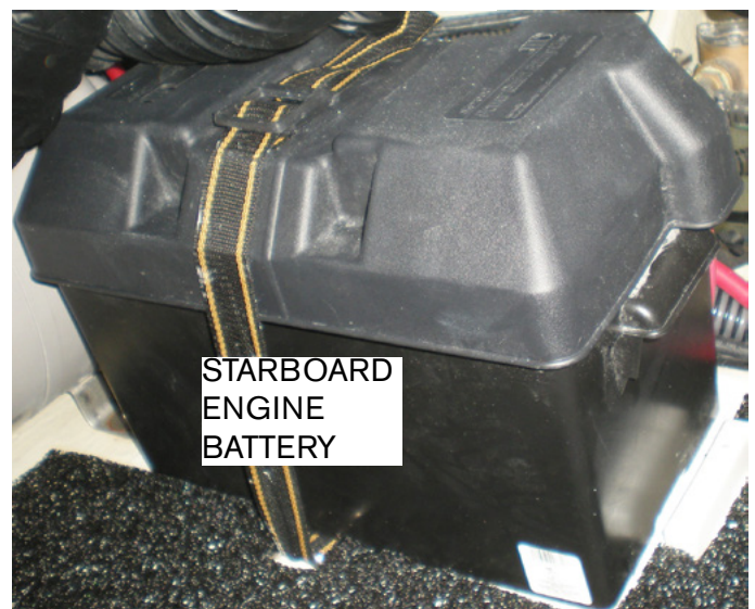
STBD AFT DECK
