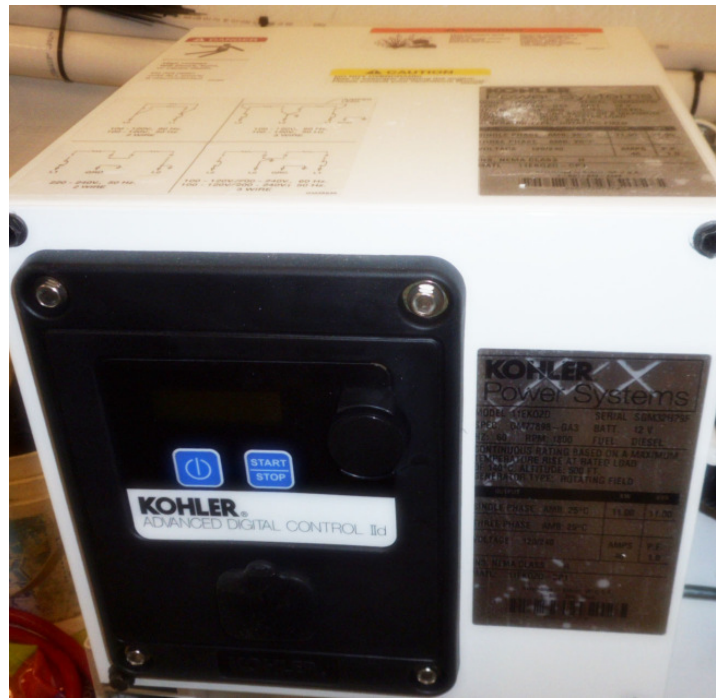
TYPICAL GEN-SET REMOTE ELECTRICAL PANEL
