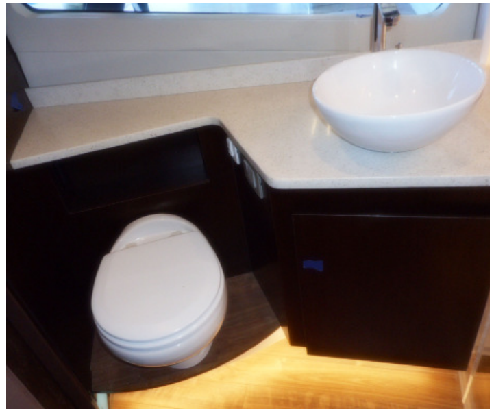
Typical Head w/ Vacuum Toilet & Vessel Sink
