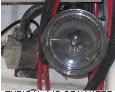
TYPICAL A/C SEAWATER STRAINER/BASKET
