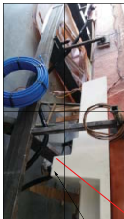
Deck Liner Drain Hose Size: Ø 1 1/2\"/>
