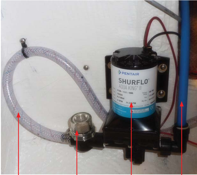
FILL HOSE FILTER STRAINER PUMP FEED HOSE
