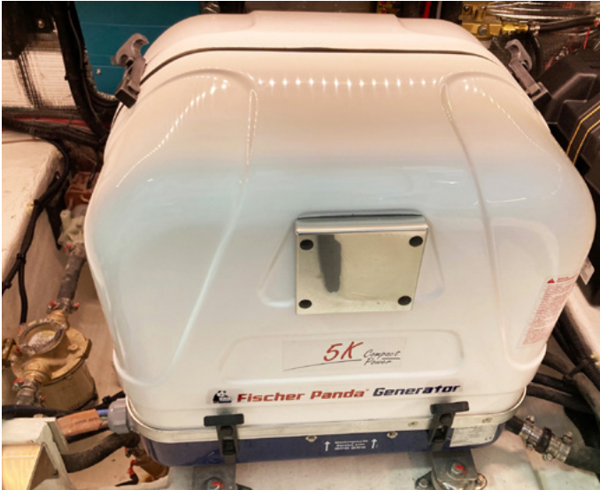
GEN-SET W/ SOUND INSULATION CAPSULE
